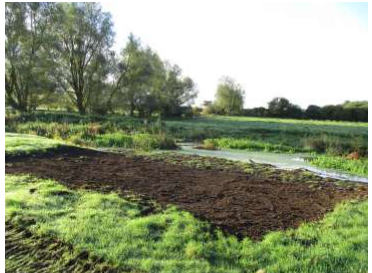
Bank re-profiling with excavator
