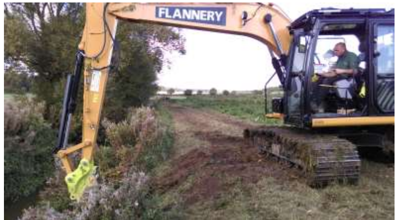
Using the excavator to key wood into the bank.
