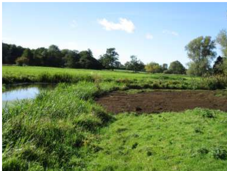
Re-profiling work completed
