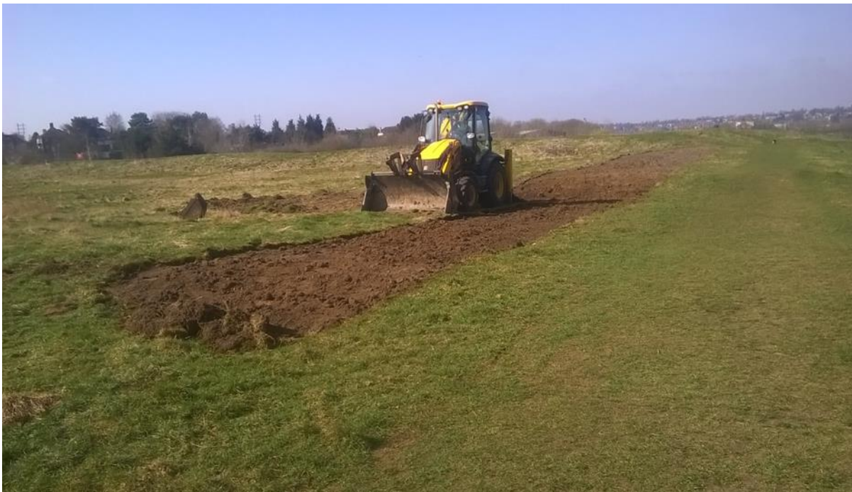
Turf stripping at Landseer Park using an excavator.
