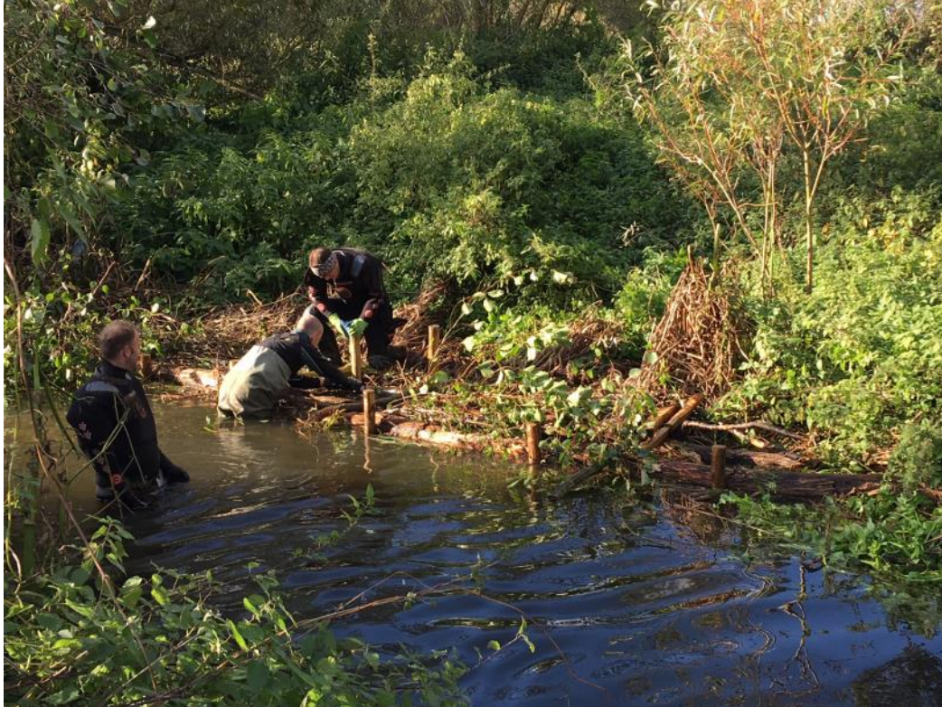
Installing features on the River Gipping
