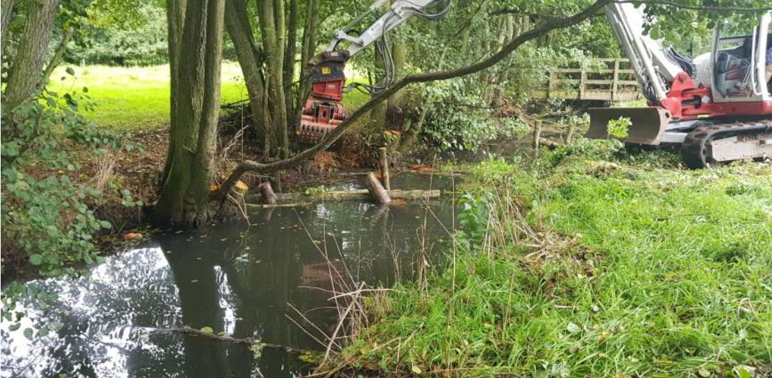
Installing a flow deflector on the River Blyth © Alice Wickman
